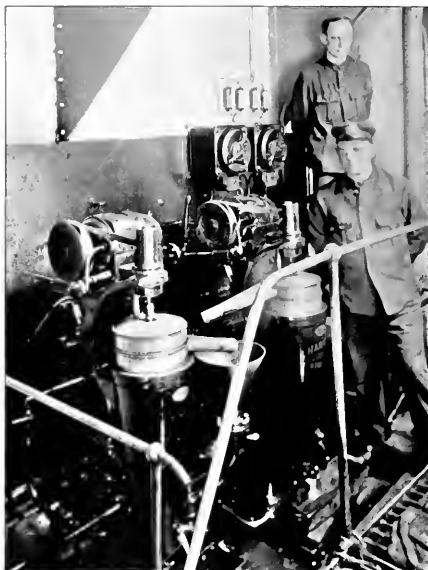
One of the interesting visitors to San Francisco harbor during the past month was the British motorship Pacific Shipper. An excellent view of this Furness, Withy freighter alongside her dock is shown below; above is view of her engine room showing two Sharples supercentrifuges installed to take care of the clarifying of fuel oil and lubricating oil used in the main engines.
